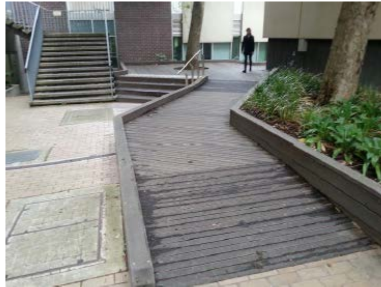
Walk down the decking
